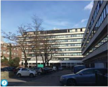
2 Building C from commercial car park
