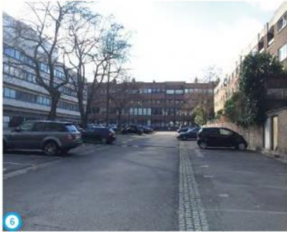
6 Building A from commercial car park
