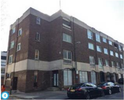
4 Building B from Blandford Street
