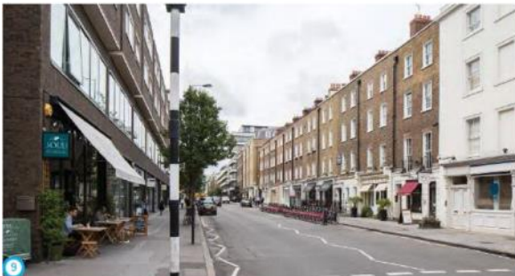
9 Building C and D from George Street
